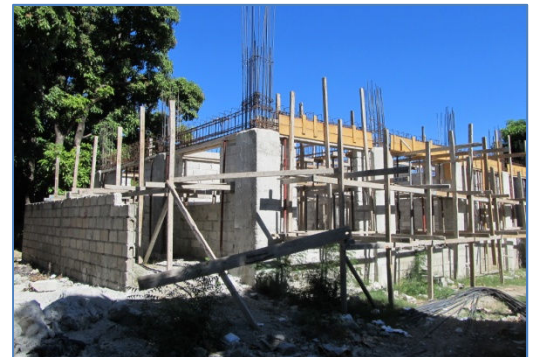
Clinic under construction
