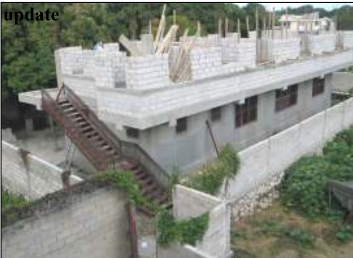
View of Patti's School second floor going up
